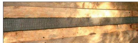
Figure 4.8 Reinforcement placed over the mortar
